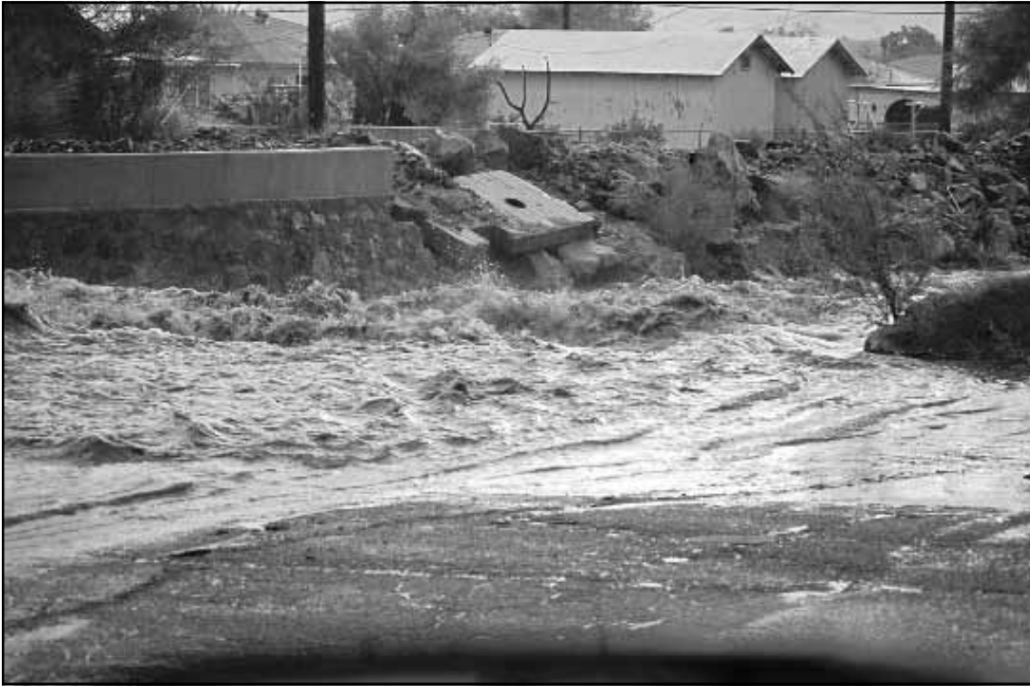
The road washed out on Cedar near the Presbyterian Church.
